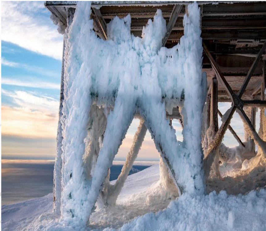
LONG RANGE RADAR SITE
